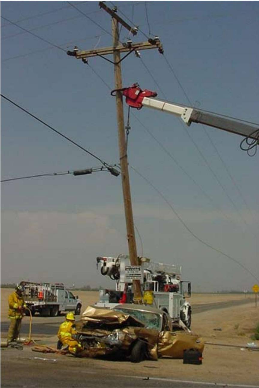
*Realize that a damaged power line or pole may drop power lines at another location out of immediate view.*
