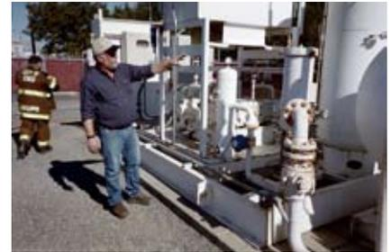
*From the pipeline natural gas is scrubbed, dried, and compressed before it is pumped to the customers vehicle.*
