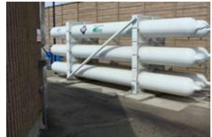
*Cylinders come in a variety of construction materials; steel, aluminum, and fiber wrapped.*
