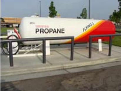
*Unlike CNG fueling stations, LPG fueling stations require a trained technician to transfer fuel to the vehicle.*
