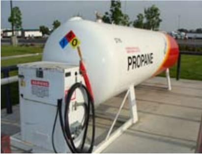
Refueling stations that offer propane are easily identified with above ground storage tanks.
